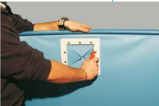
Then use a wallpaper knife to cut the liner inside the flange so that the skimmer opening is free.
