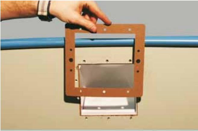
Take the second seal and position it on the inside of the steel jacket.
