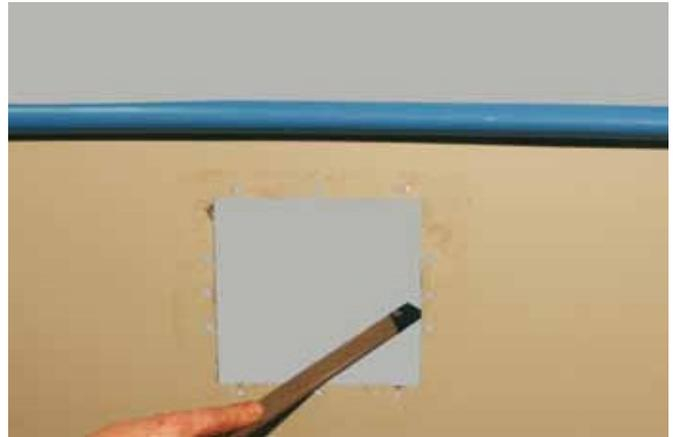
Deburr the sheet metal with a file so that there are no sharp edges.
