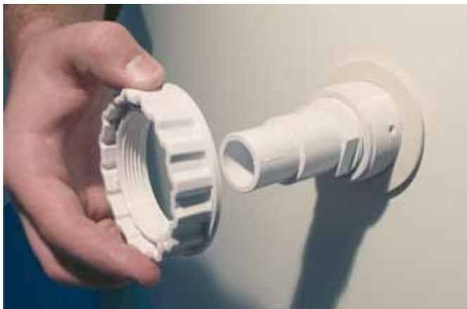
Take the lock nut, place it on the nozzle from the outside, and tighten it by hand.
