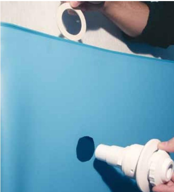
Now place a seal on the nozzle and push the nozzle through the hole from the inside to the outside.
