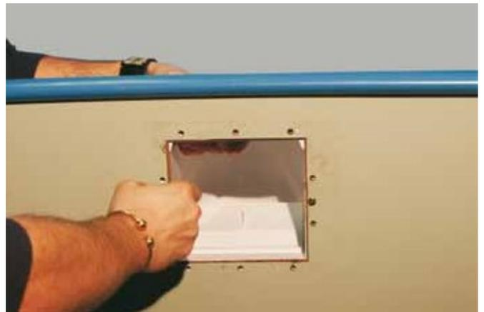
Screw the skimmer firmly to the steel wall on the right and left using two of the screws provided.
