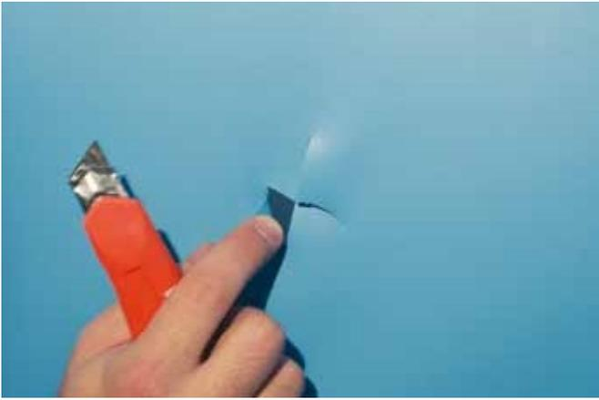
The intended position for the nozzle is already stamped into the steel sheet casing.
