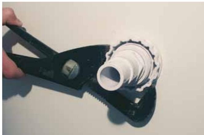
Now you can carefully tighten the lock nut with pliers.
