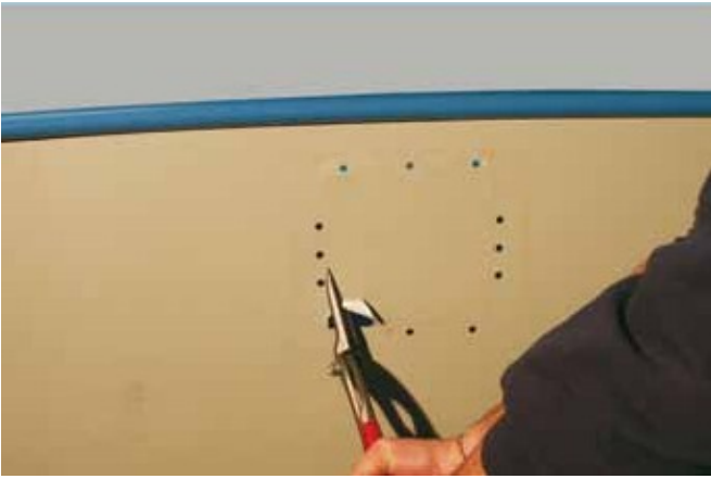
Cut out the skimmer opening with tin snips.
