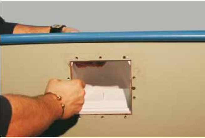
Screw the skimmer firmly to the steel wall on the right and left using two of the screws provided.
