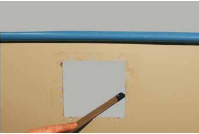
Deburr the sheet metal with a file so that there are no sharp edges.
