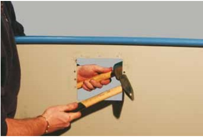
If the sheet metal has become slightly deformed, you can tap it into shape with two hammers.
